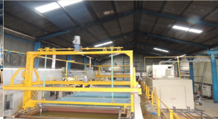
CED COATING PLANT, JAMSHEDPUR
