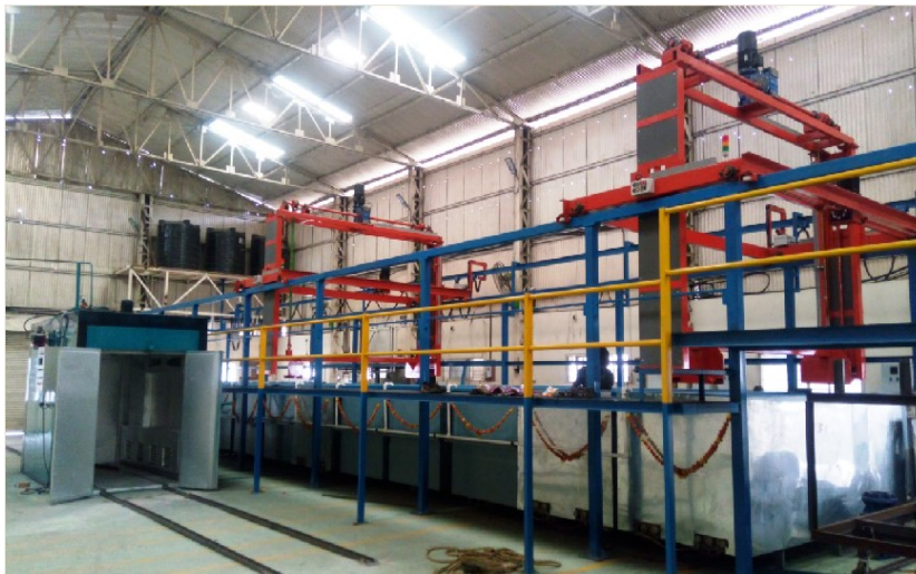
CED COATING PLANT, PUNE
